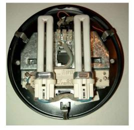
**Figure 10** One ballast suffices for two smaller lamps, reducing the levels of both reactive power and active losses below the level which otherwise one lamp alone would cause
